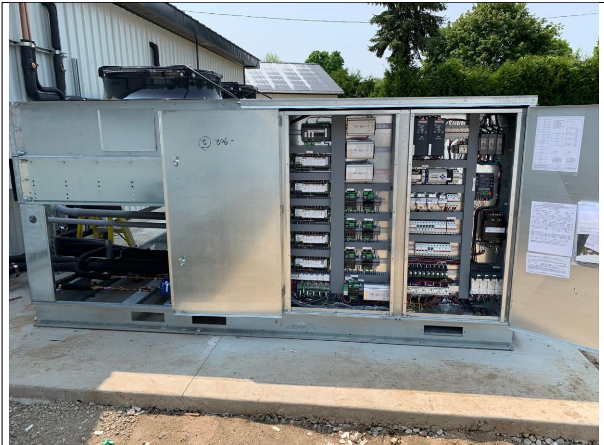
Figure 10 – System Controls – No Mechanical/Electrical Room Required
