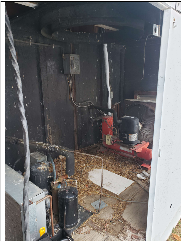
Figure 1 – Base Case Freezer Systems
