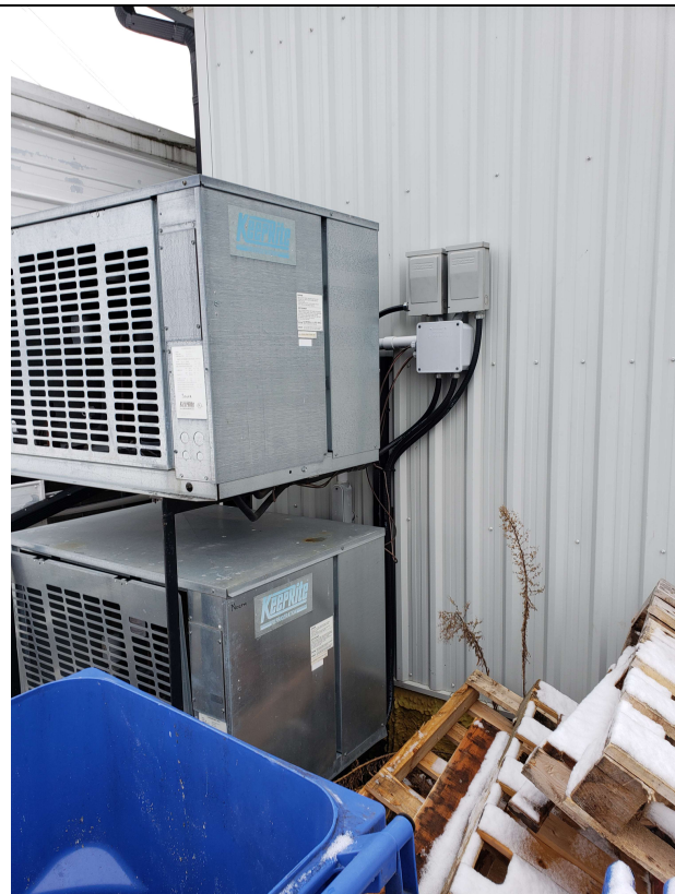
Figure 2 – Base Case Cooler Systems
