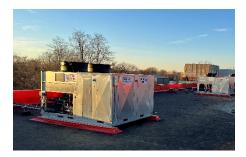
at considerably higher pressures than HFO low-pressure refrigerants. Higher pressures can cause stress on system components, resulting in greater maintenance requirements. The option of using an environmentally friendly low-pressure refrigerant combined with a system designed to eliminate the need for high pressures and mechanically driven components can provide a solution with longevity.
